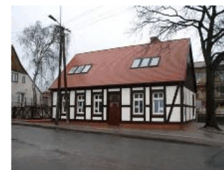
13, Kosynierów Street after rehabilitation
