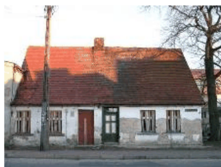
13, Kosynierów Street before rehabilitation
